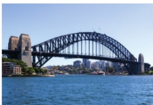
The girders of the Sydney Harbour Bridge demonstrate alternate angles and parallel lines.
